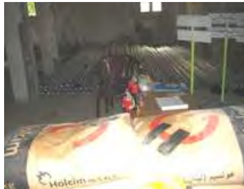
2. Project materials – pipes, valves, fittings & cement in locked storage.
