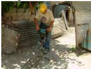
4. Breaking ground with jack hammer.
