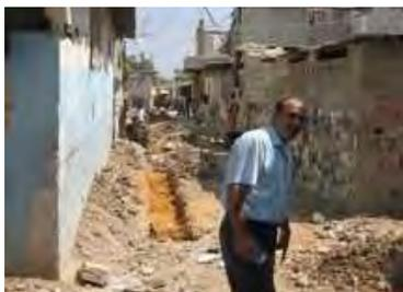
10. Newly installed pipes protected with coarse sand.
