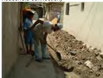
11. Backfilling trench over coarse sand.
