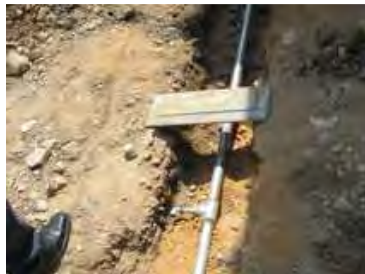
8. ¾" pipe in trench (from main pipe to household connection)
