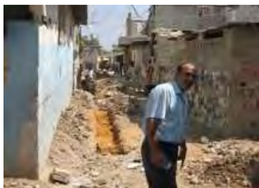
10. Newly installed pipes protected with coarse sand.
