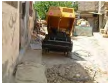
5. Compressor for jack hammer.
