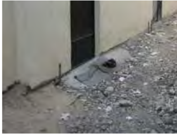
13. Backfilled trench in foreground and individual household connection upstands beside wall.
