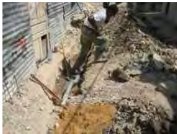
7. 3" diameter main pipe in trench
