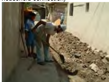
11. Backfilling trench over coarse sand.
