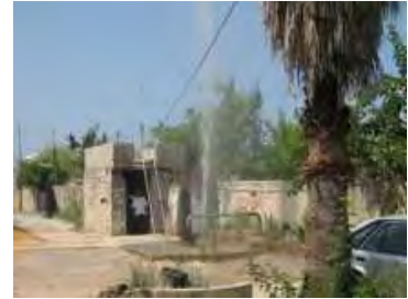
15. Testing water pressure at well head.
